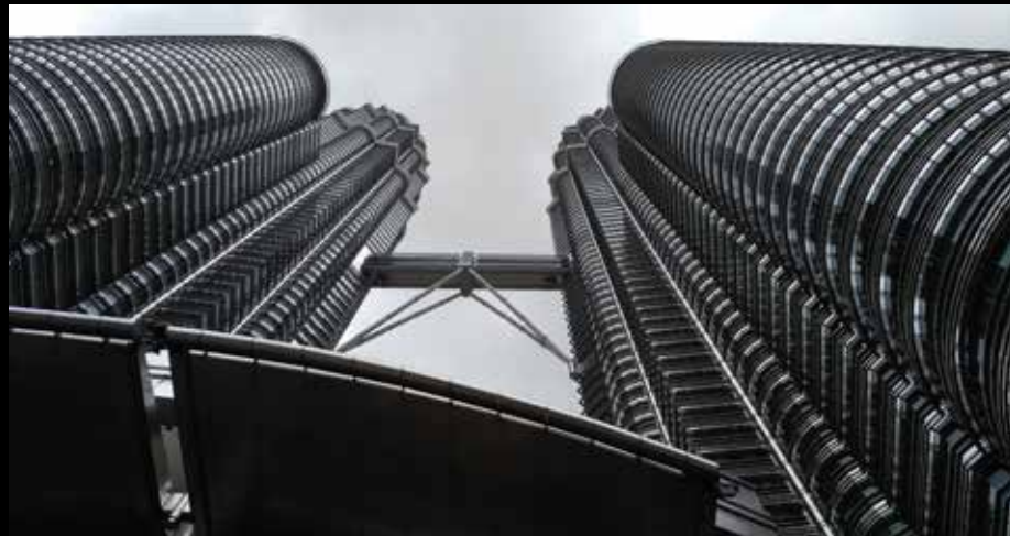
FIGURE 6: Petronas Twin Towers skybridge connects both towers with three functions –symbolism, structural soundness and safety
